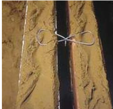
Fig 2 - Wall tie installation
