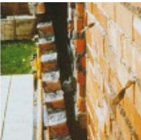
Fig 5 - Separation of outer leaf
