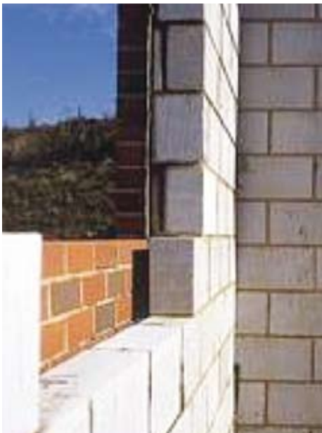
Fig 1 - Modern brick / block cavity wall
